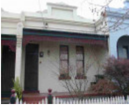
clifton hill fenwick street clifton hill fenwick street 33
