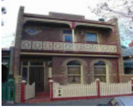
clifton hill fenwick street clifton hill fenwick street 34
