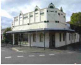
clifton hill fenwick street clifton hill fenwick street 40
