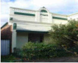
clifton hill fenwick street clifton hill fenwick street 44
