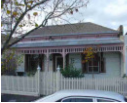
clifton hill fenwick street clifton hill fenwick street 46
