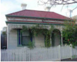
clifton hill fenwick street clifton hill fenwick street 50
