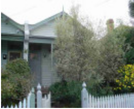
clifton hill fenwick street clifton hill fenwick street 51
