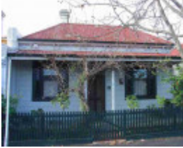
clifton hill fenwick street clifton hill fenwick street 52
