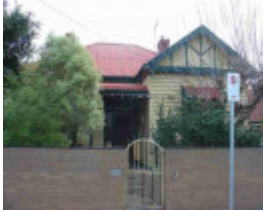
clifton hill fenwick street clifton hill fenwick street 53
