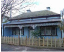
clifton hill fenwick street clifton hill fenwick street 58
