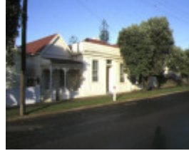
1 former builders inn portland street view aug1985
