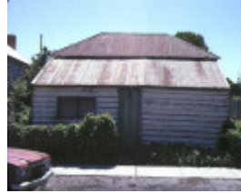
1 dwelling 8 glenelg street portland front view
