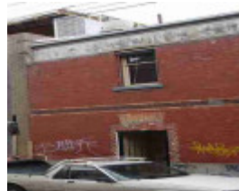
fitzroy argyle street fitzroy argyle street 20-26
