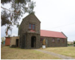
FORMER NATIONAL SCHOOL SOHE 2008
