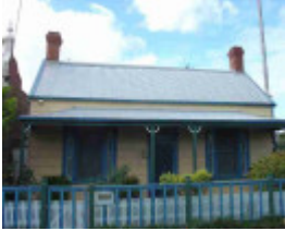
clifton hill fenwick street clifton hill fenwick street 2
