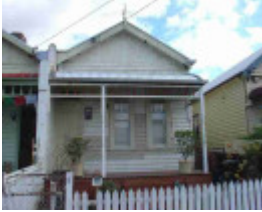
clifton hill fenwick street clifton hill fenwick street 5
