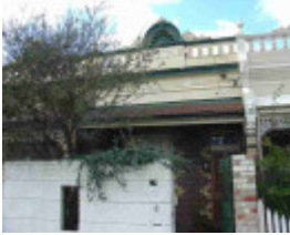
clifton hill fenwick street clifton hill fenwick street 6
