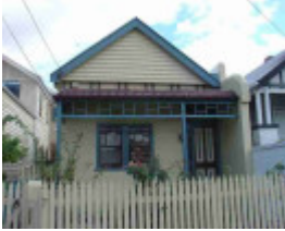
clifton hill fenwick street clifton hill fenwick street 7
