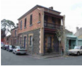
fitzroy argyle street fitzroy argyle street 99
