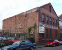
fitzroy argyle street fitzroy argyle street 25 unit 1
