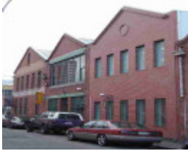
fitzroy argyle street fitzroy argyle street 29-31
