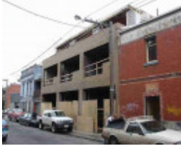
fitzroy argyle street fitzroy argyle street 30-34
