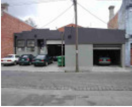
fitzroy argyle street fitzroy argyle street 44
