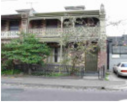
fitzroy argyle street fitzroy argyle street 48
