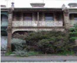
fitzroy argyle street fitzroy argyle street 50
