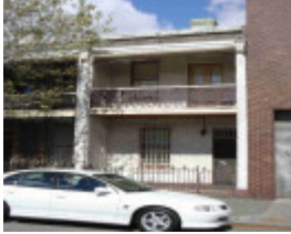
Fitzroy Kerr Street 76.JPG
