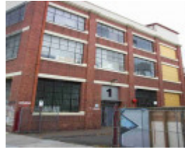
Clifton Hill Parslow Street 1 v2.JPG
