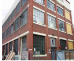
Clifton Hill Parslow Street 1 v3.JPG
