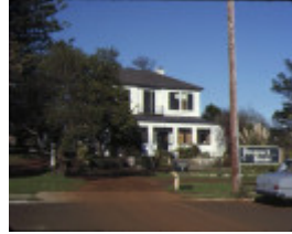
1 prospect portland front view from street
