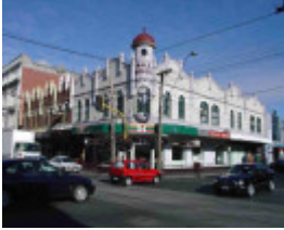
Fitzroy Brunswick Street 287-295.JPG
