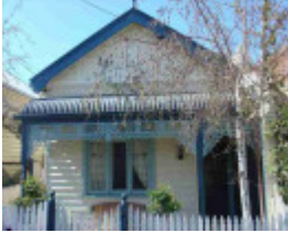
clifton hill kiewa street clifton hill kiewa street 10
