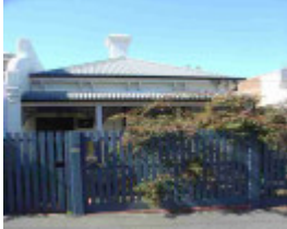
clifton hill kiewa street clifton hill kiewa street 16
