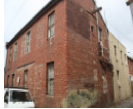
Rear of 78 Nicholson Street.JPG
