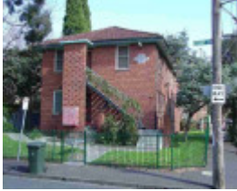
fitzroy fitzroy street fitzroy fitzroy street 207 unit 1
