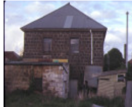
1 jay's laundry portland rear view
