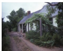
belmont raglan road beaufort side view homestead mar1985
