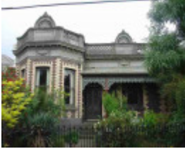
fitzroy north holden street fitzroy north holden street 11
