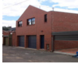
Rear of 31 Arnold Street.JPG
