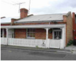
fitzroy chapel street fitzroy chapel street 39
