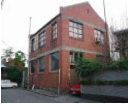
fitzroy chapel street fitzroy chapel street 40
