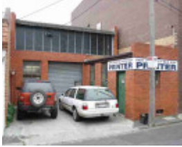
fitzroy chapel street fitzroy chapel street 41
