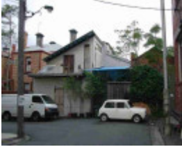
fitzroy chapel street fitzroy chapel street 42
