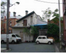
fitzroy chapel street fitzroy chapel street 42
