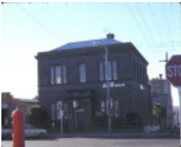
1 anz bank portland front view
