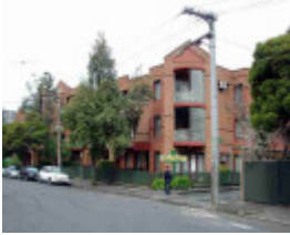
fitzroy palmer street fitzroy palmer street 28-34
