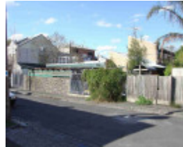
Fitzroy John Street 21-23 REAR CREMORNE Street FACADE.JPG
