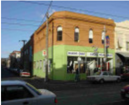
fitzroy brunswick street fitzroy brunswick street 226a-230
