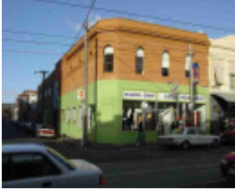
fitzroy brunswick street fitzroy brunswick street 226a-230
