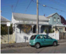
richmond durham street richmond durham street 3
