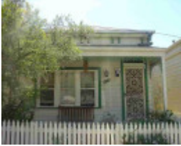
clifton hill kiewa street clifton hill kiewa street 22
