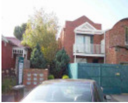
clifton hill noone street clifton hill noone street 146 unit 7
