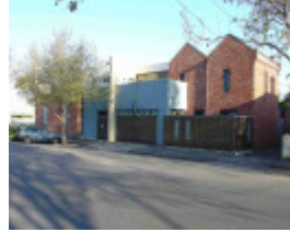
Fitzroy Napier Street 423 Westgarth Street FACADE.JPG
