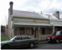
fitzroy argyle street fitzroy argyle street 109
